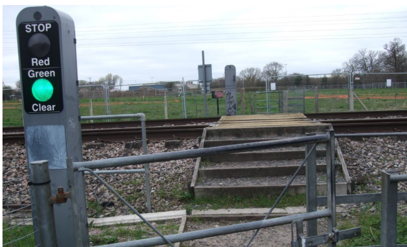
Level crossing is unaltered
